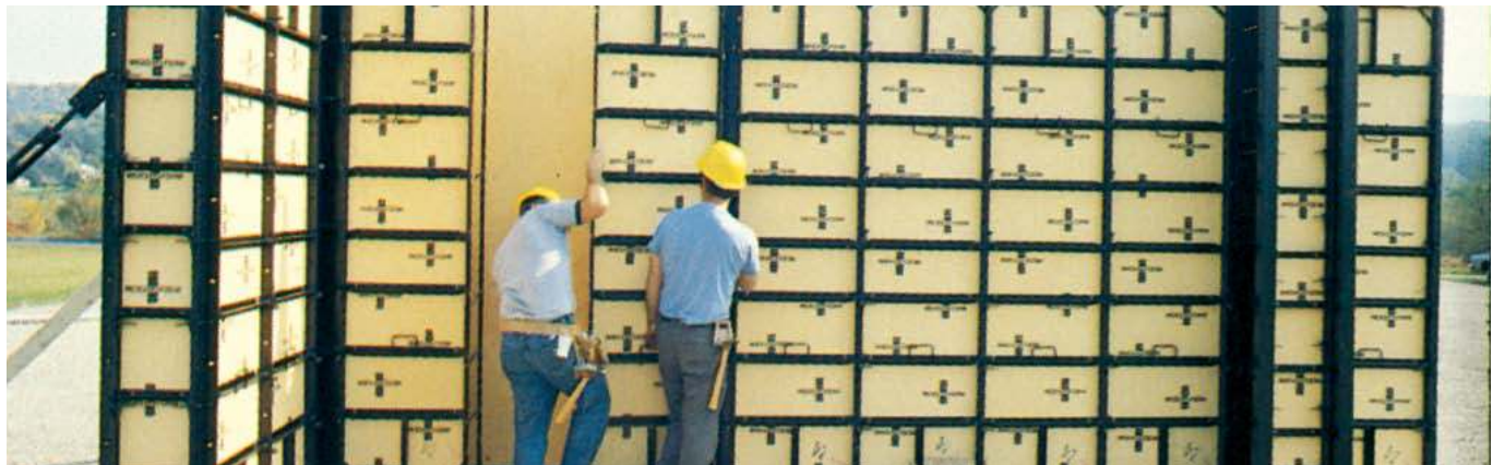
MOD-U-FORM Highly productive, heavy-duty plywood-faced, steel encased panels offer unlimited versatility in forming structures that can be straight, curved, haunched, round, battered or angled.
